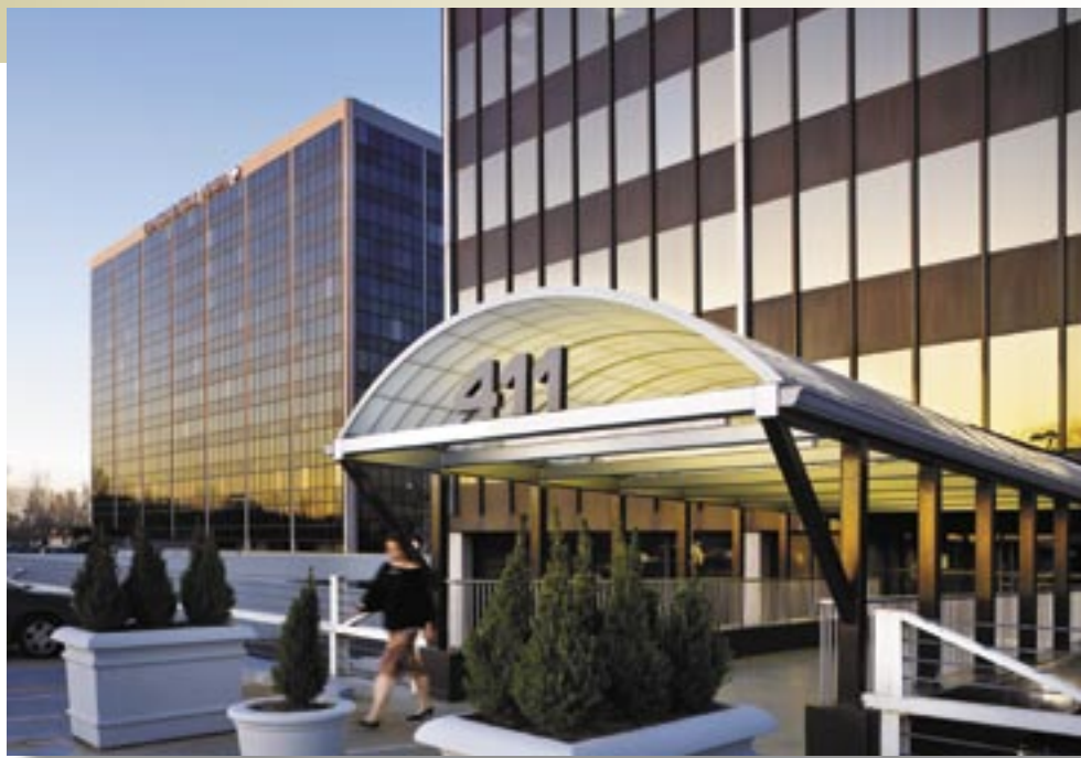
Continental Plaza's new canopies, one the many complex upgrades
