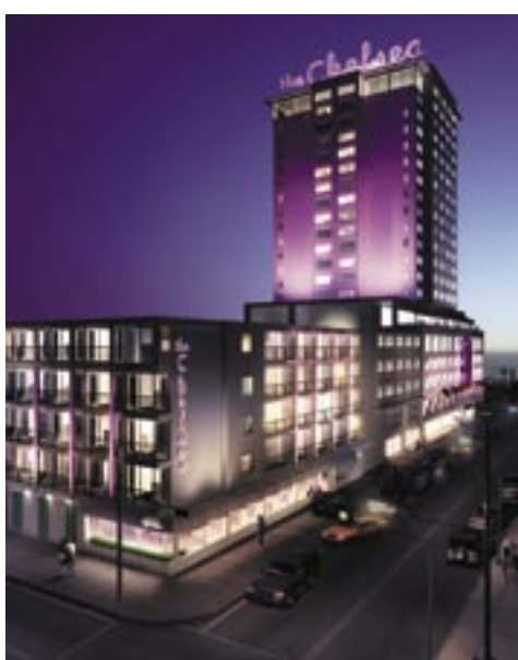
Newly renovated Chelsea Hotel, Atlantic City, New Jersey
